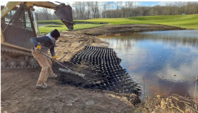
*Figure 9. Pond bank stabilization products should be installed where possible to prevent bank erosion.*
