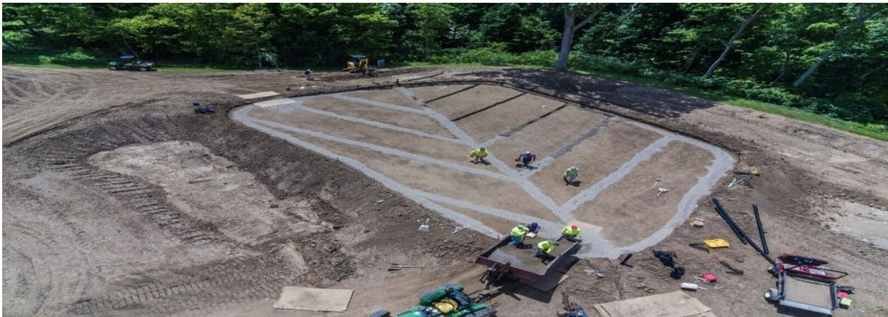
Figure 3. When constructing drainage systems, pay close attention to engineering details such as subsoil preparation, the placement of gravel, slopes, and backfilling. Photo credit: Jason Mahl.
