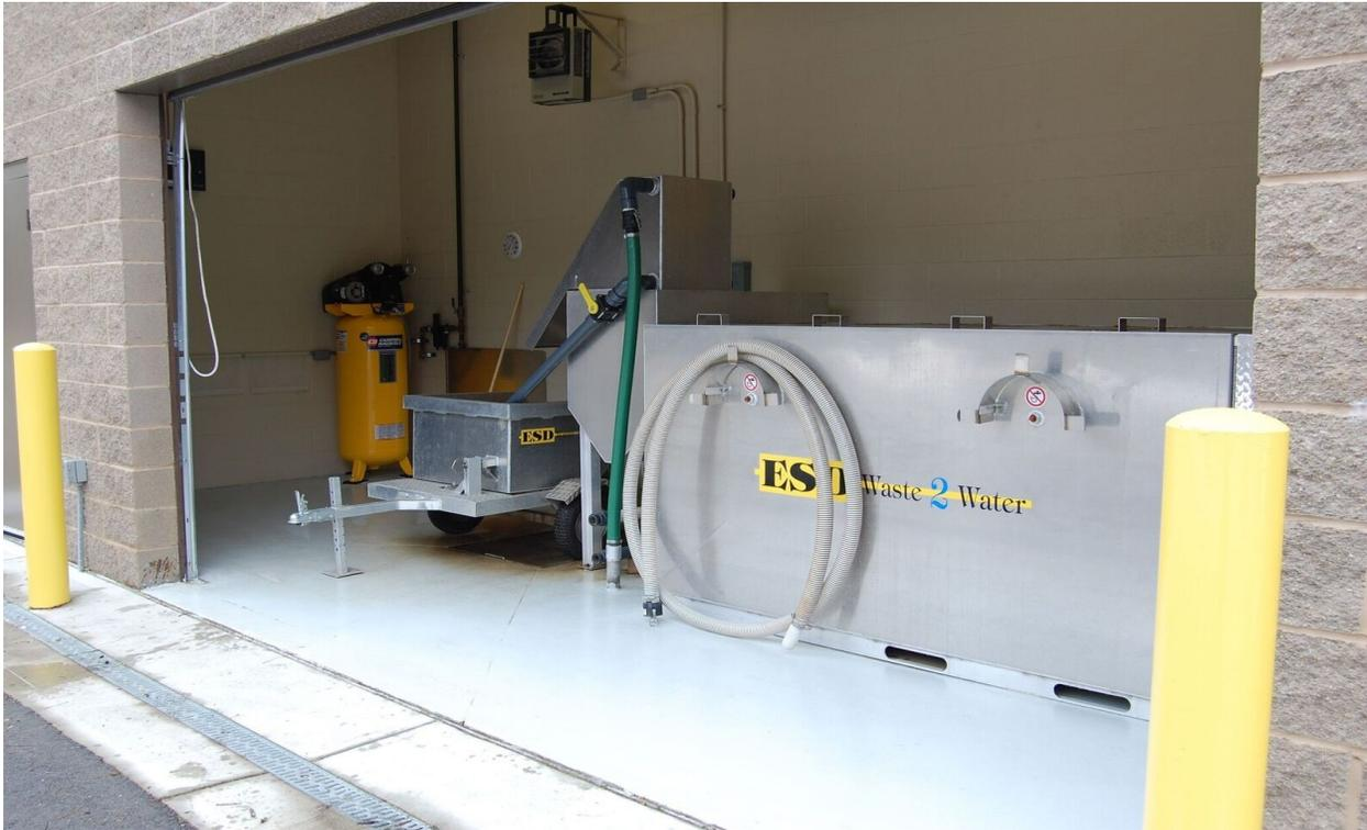
*Figure 33. Wash equipment over a concrete or asphalt pad that allows the water to be collected. Photo credit: Jason Mahl.*
