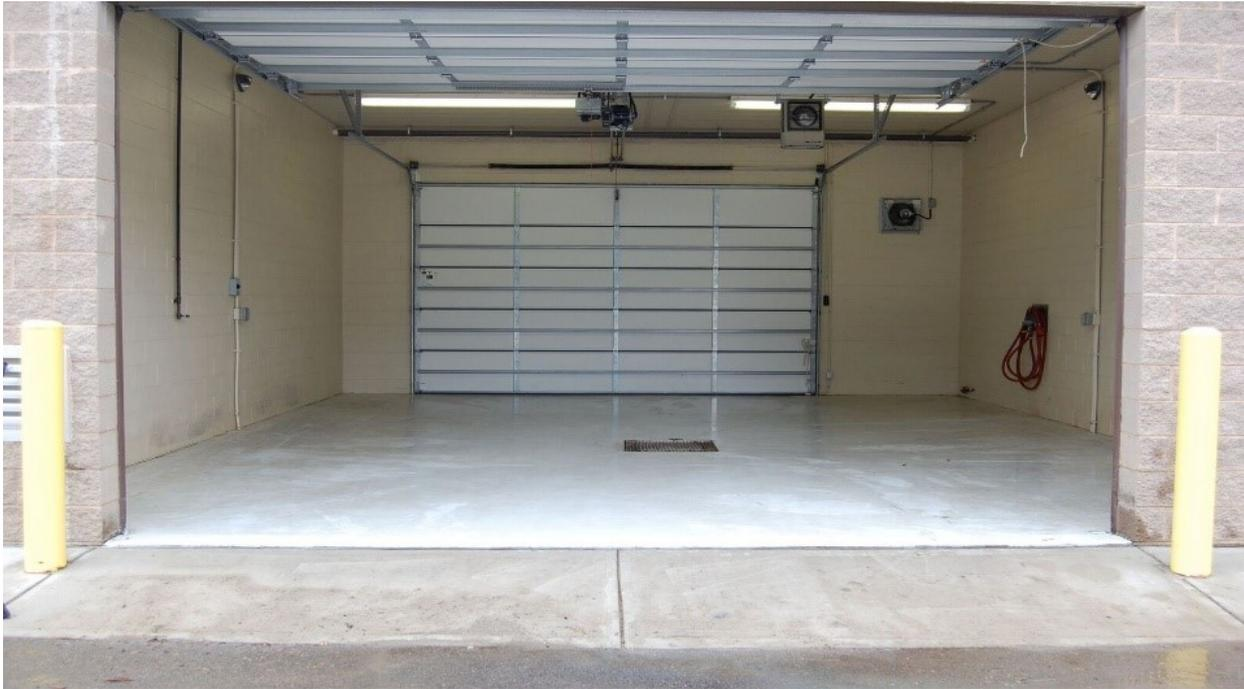
*Figure 4. Construct floors of seamless metal or concrete sealed with a chemical-resistant paint. Photo credit: Jason Mahl.*
